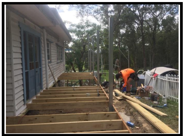
Steel post and sub floor construction as at May 2018.
