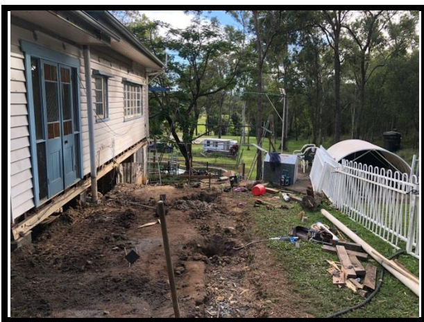
Set out and footing stage of wrap around verandah and decks in Gilston.
