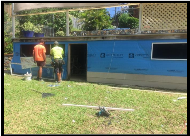
Replacement of timber framing and fibre cement cladding 2016.
