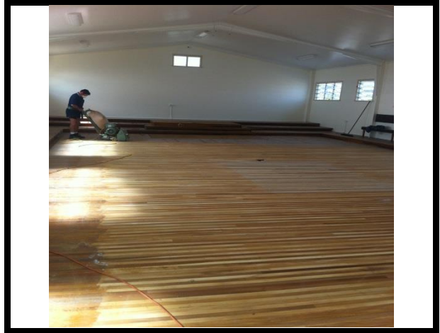
Sanding back to re-polish timber floors in the Freemasons Lodge, Tully QLD.
