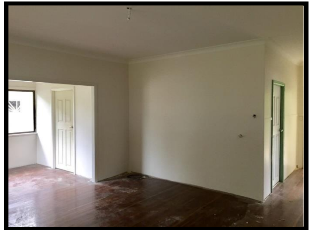
New plaster board wall and ceiling linings. Light sand and re-polish of timber floors next stage.
