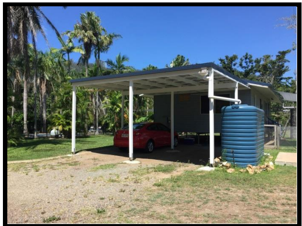
Completed carport, hardwood post, beams, rafters and battens construction.
