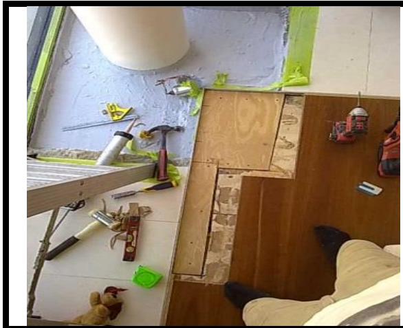
New base and ply underlay installed.
