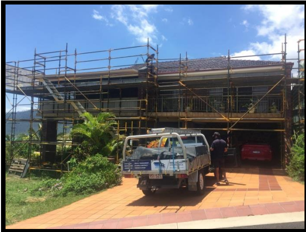
Scaffold erected for tile roof replacement, 2018.
