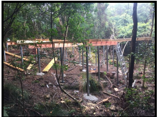
Bearers and floor joist construction stage.
