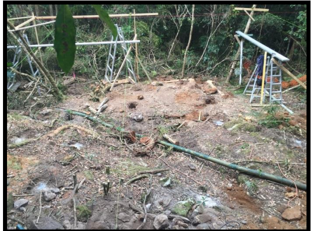
Setting out building location, steel post positions.
