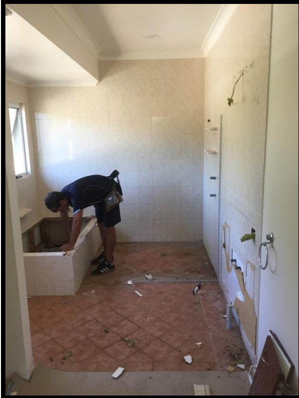
Demolition stage of a bathroom renovation. Moving shower to bath location and new door in showers place on right hand wall, 2016.
