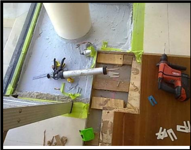
Removal of water damaged timber floor Sovereign Island, 2014.
