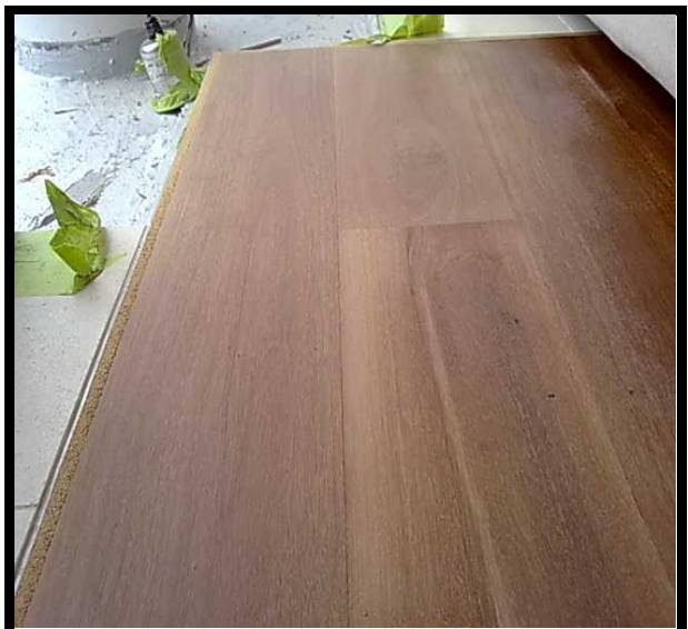
Cork expansion joint installed. Ready for sand and polish.
