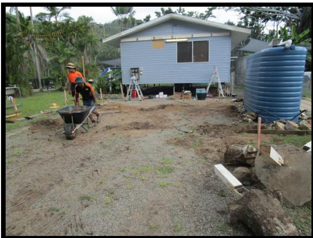
Existing carport removed. Footing and set out stage 2017.
