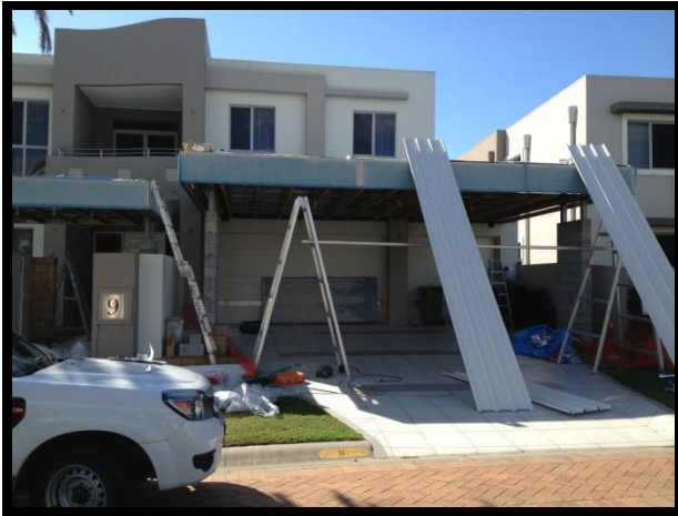
Roofing stage, clip lock roofing used.
