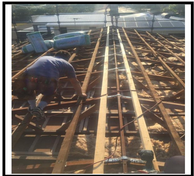
Upgrade of roof frame to today's standard.
