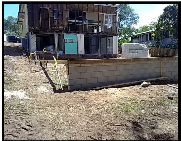
Footing and block wall constructed, slab preparation stage in Redhill.
