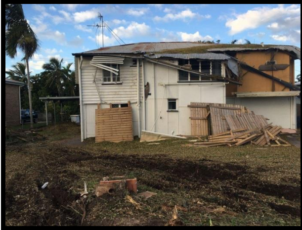
Mackay house damaged by falling tree. Make safe included asbestos removal and decontamination 2017.
