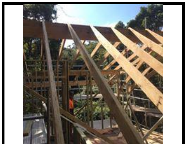
Hand pitching roof rafters.
