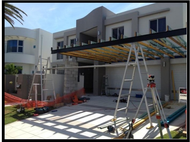
Construction stage showing block piers, steel beams, posts and trusses.
