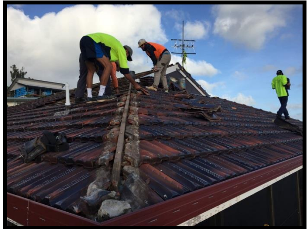
Work beginning on tile roof replacement.
