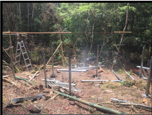
Installing steel posts to bedrock and or pier footings.
